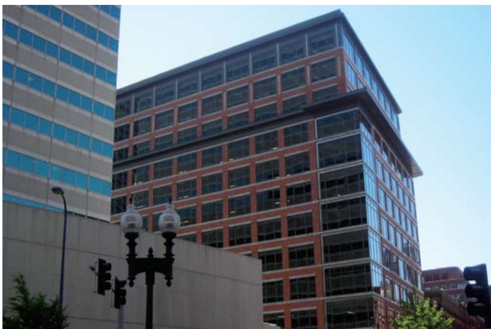
TWO FINANCIAL CENTER IS A MAJOR PROJECT IN BOSTON, ON TRACK FOR COMPLETION IN 2009.
